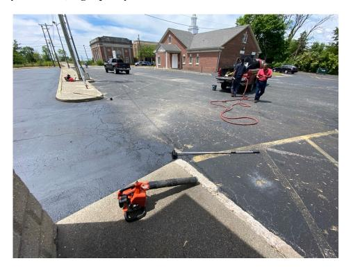
The picture above is an example of a poor quality seal coating project. The contractor is using a small handheld blower to prepare the parking lot (Prep is the most important part of the job), dirt and cracks are visible yet they are still sealcoating the parking lot using a square tank in the back of a pickup truck.
