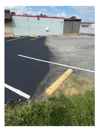
The picture above is an example of a poor quality seal coating project a customer received from not properly qualifying a seal coating contractor.
