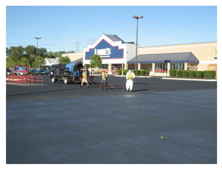
In this verification picture it is visibly evident of the 2<sup>nd</sup> coat of pavement sealer being applied.
